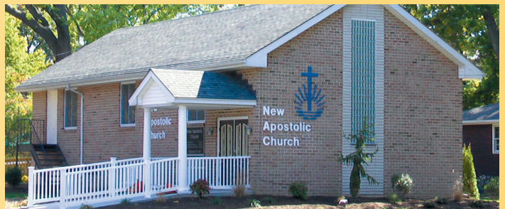
Church renovation in Cinnaminson, NJ
