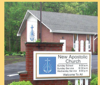
Church after renovation - Dix Hills, NY
