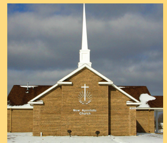
New church building in Wyoming
